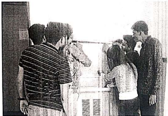
Replacement of Water Cooler Tap (QTY: 2)
